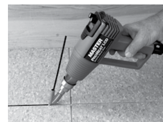
Welding Flooring Material
